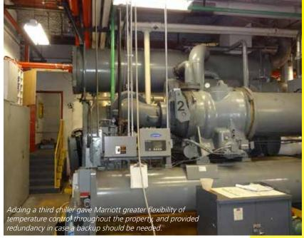
cause of the chiller size, even on a mild day, they might have needed to use both of them. Smaller equipment allows for greater flexibility in switching from one to another. It's just a better way to run the building without relying on two older pieces of equipment."
