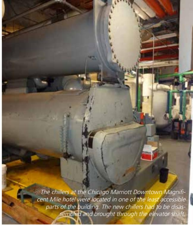
The chillers at the Chicago Marriott Downtown Magnificent Mile hotel were located in one of the least accessible parts of the building. The new chillers had to be disassembled and brought through the elevator shaft.
