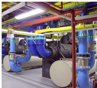
Chilled water distribution will be inefficient if temperature differentials don't match design parameters. Check out our tips for avoiding, identifying, and fixing this problem, also known as "Low  $\Delta T$ " or "Low Delta-T" syndrome.
